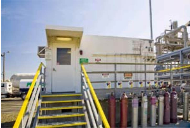
Carbon dioxide is piped into the quality assurance building from the purification plant. From there it is pumped into the waiting tanker.
